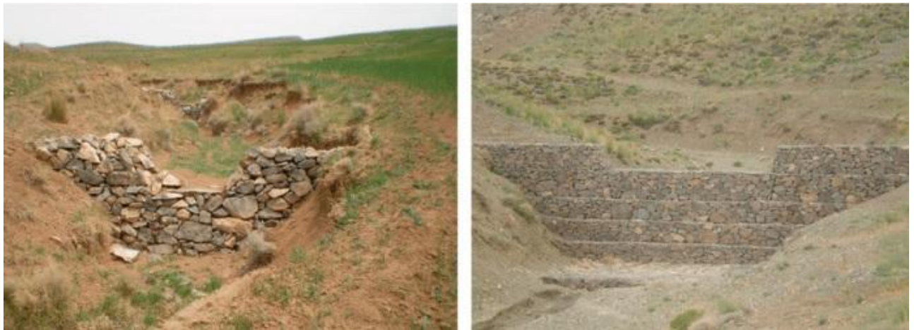
Figure 3.30: 2 examples of permeable rock dams
