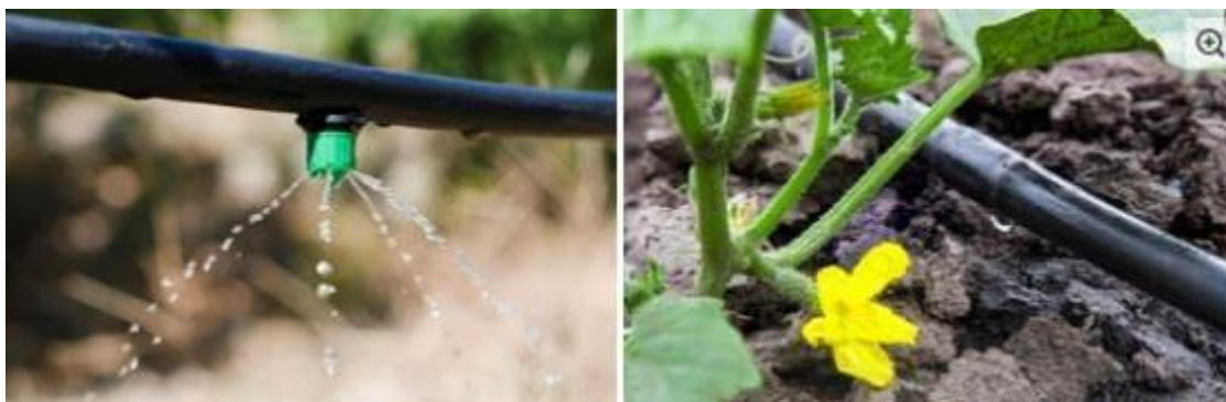
Figure 3.35: Overhead plastic pipe with drip emitter and a ground drip system (Impuls Africa)
