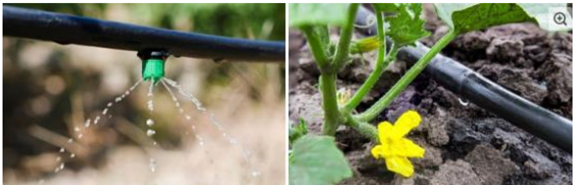
Figure 6.3: An Overhead Plastic Pipe with Drip Emitter and a Ground Drip System
